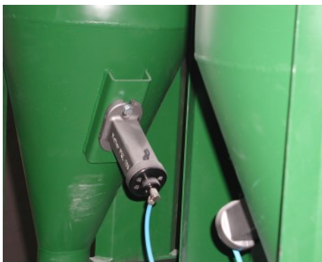
PKL 450 mounted on the cone of a granulate hopper
