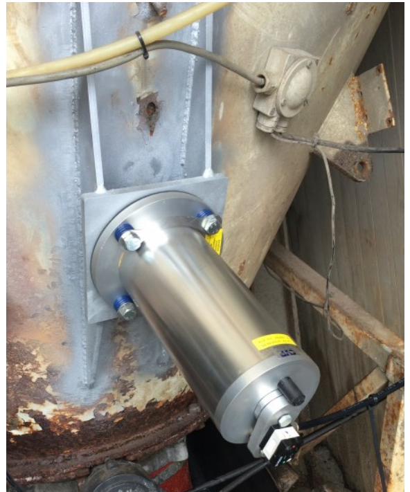
PKL 2100 with ASB bracket installed on a silo outlet
